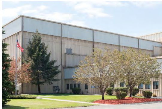
Figure 9. The Ramsey/Washington Recycling & Energy Board owns the Recycling & Energy Center, a refuse derived fuel processing facility in Newport, Minnesota.
