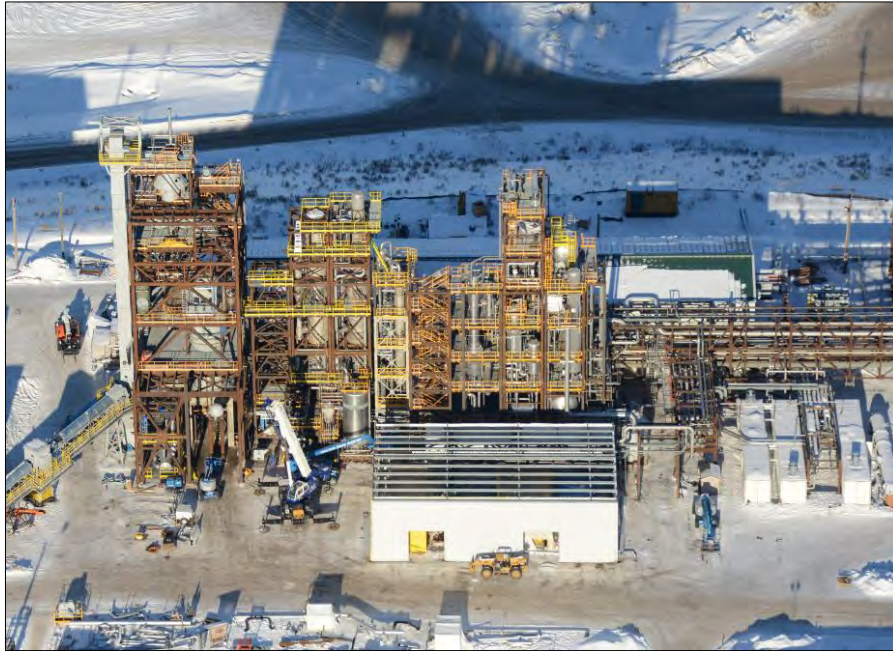
Figure 4-7 World's First Full-Scale MSW-to-Biosolids Facility Edmonton, Alberta (Canada)
